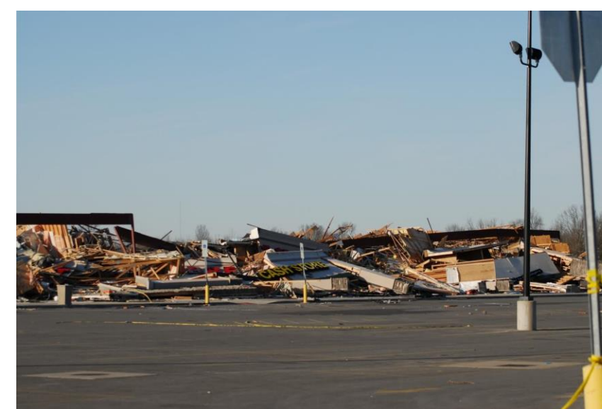
Top: Strip Mall at U.S. 45 & U.S. 145 in Harrisburg, IL destroyed
